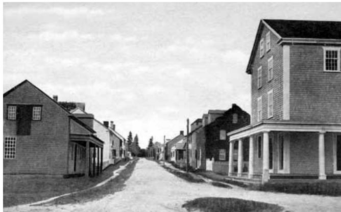
Looking north at foot of Main Road at the Cory store
