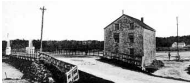
Westport Point bridge along with Lees wharf built by Thomas Mayhew c.1830
