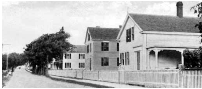
Looking north around 1958 Main Road
