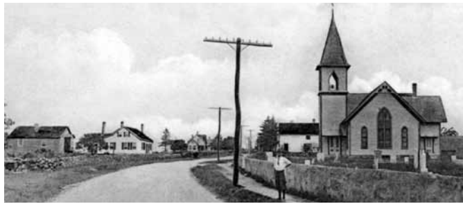
Main Road view north, note taller steeple on the Methodist Church
