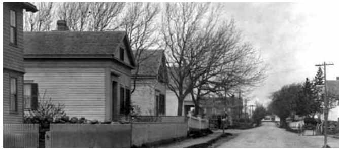
Looking north around 1973 Main Road
