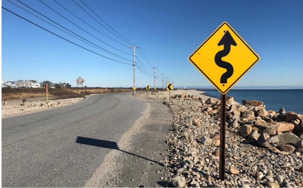
Figure 40 Ground level view of utility poles located seaward of East Beach Road.
