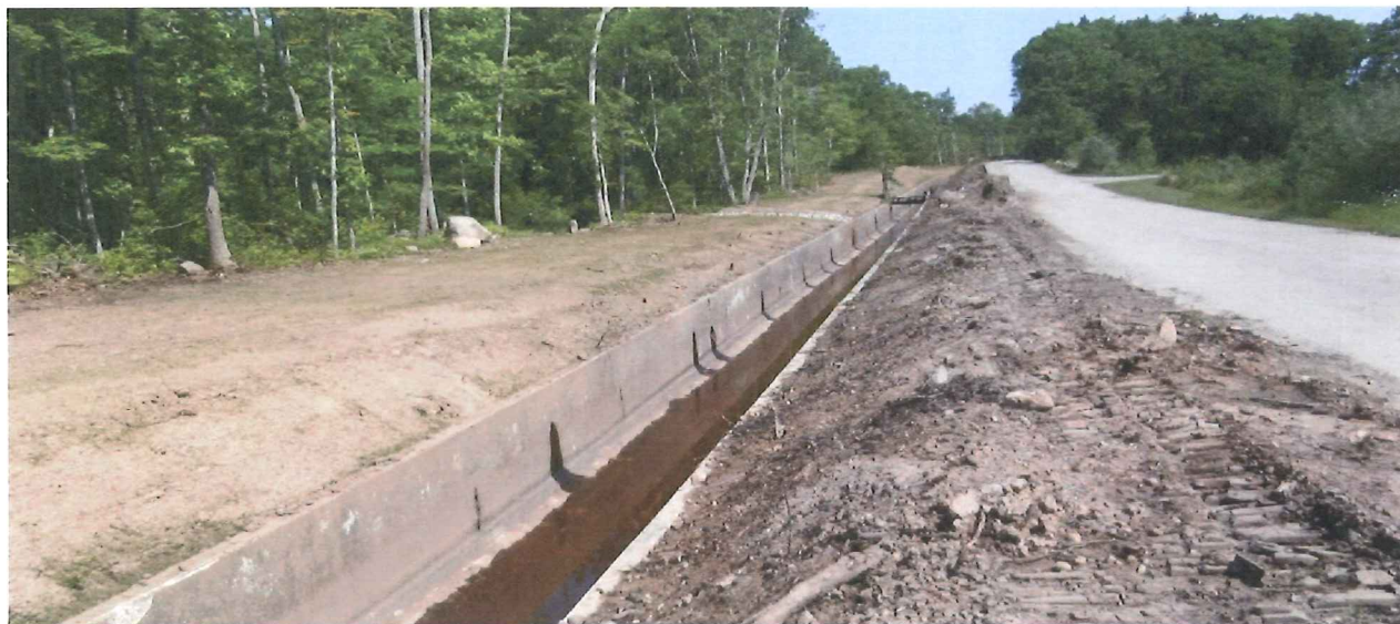
INTERCEPTOR DRAIN, AFTER TREE REMOVAL
