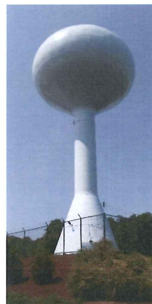
WATER STORAGE TANK AIRPORT RD
