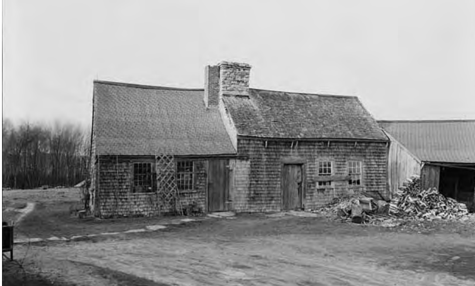
Figure 1.10: The house in 1934. HABS, Arthur C. Haskell, photographer, General view from southwest, HABS MASS, 3 WESPOS, 1-1.
