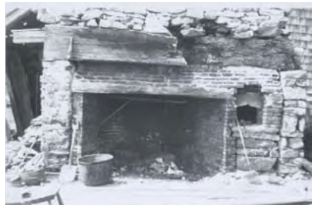
Figure 4.14: Historical photograph of the stone chimney, facing west, with intact smaller brick firebox and bake oven, date unknown, but post 1954. Courtesy of Muriel Bibeau.
