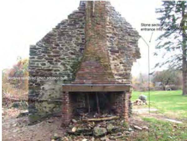
Figure 5.3: Anne Baker's annotated photograph of the west side of the stone chimney showing evidence of the original beehive oven (Courtesy of Anne Baker, 2009).
