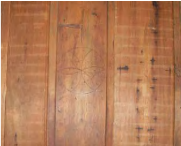
Figure 1.12: Compass carvings and lath/plaster marks on reused board sheathing currently in the Wilbor House in Little Compton, but salvaged from the Waite-Kirby-Potter house in the 1950s. (Courtesy Little Compton Historical Society).
