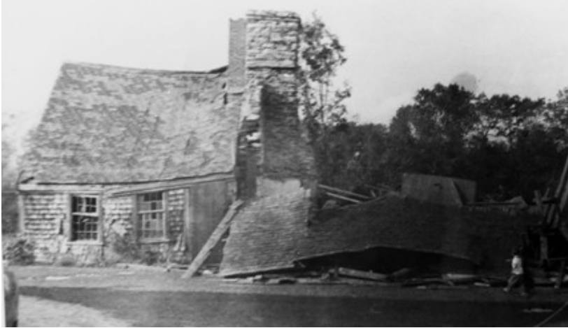
Figure 1.11: Waite-Kirby-Potter house after 1954 hurricane (Courtesy M. Bibeau).
