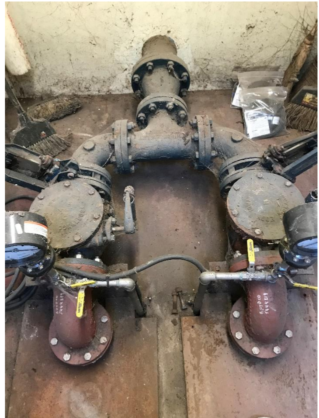
Figure 4 – White's Pump Station Exterior Access Hatch (left) and Connection of Submersible Pumps to 6" Force Main (right)
