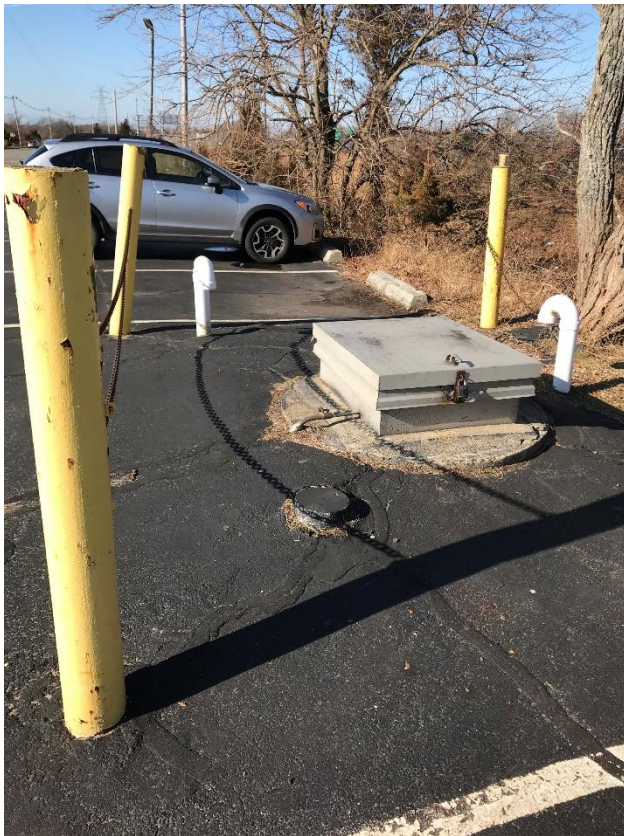
Figure 4 – White's Pump Station Exterior Access Hatch (left) and Connection of Submersible Pumps to 6" Force Main (right)
