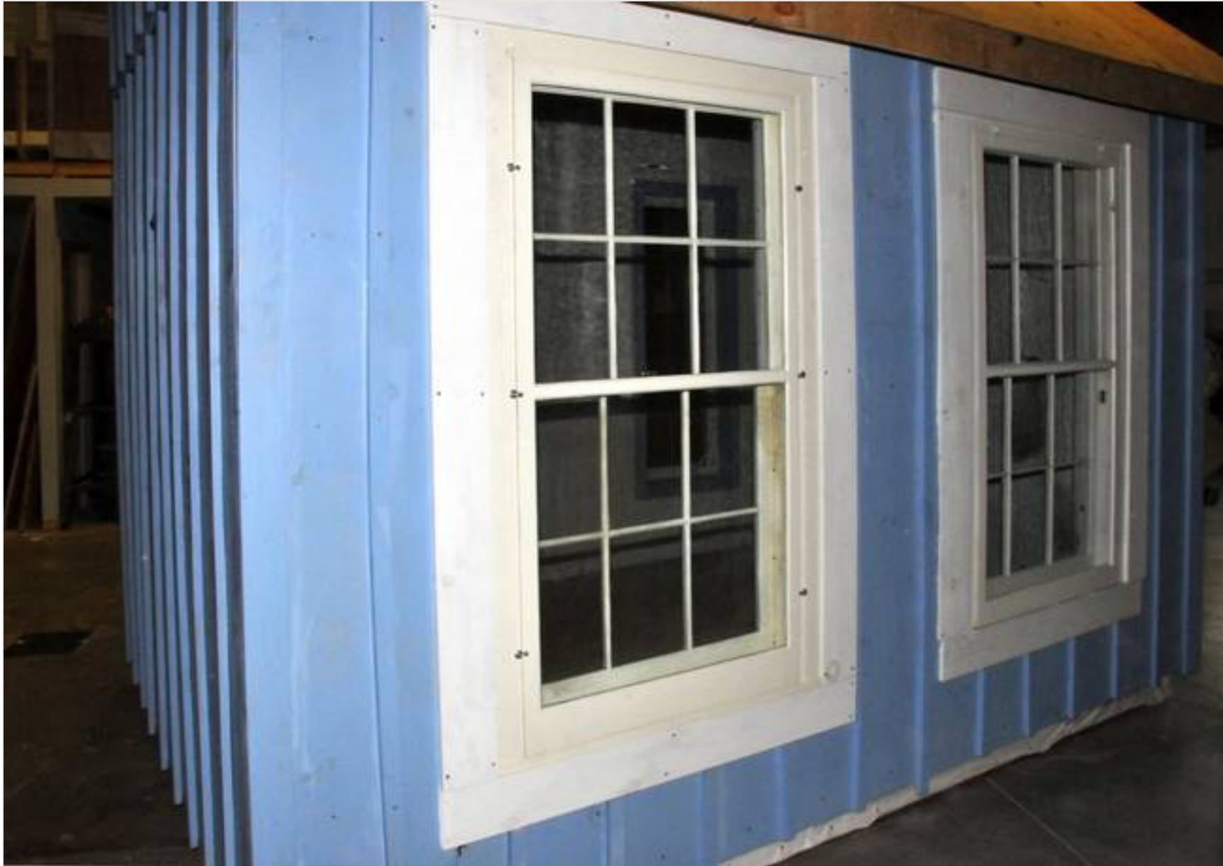
© Shannon Kyles/ Restored windows installed in tiny house
