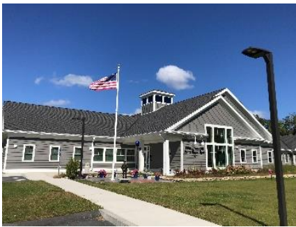
NEW POLICE STATION
