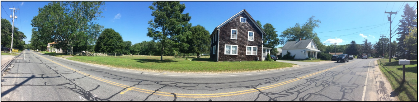
Fig. 6 - Central Village—Adamsville Road.
