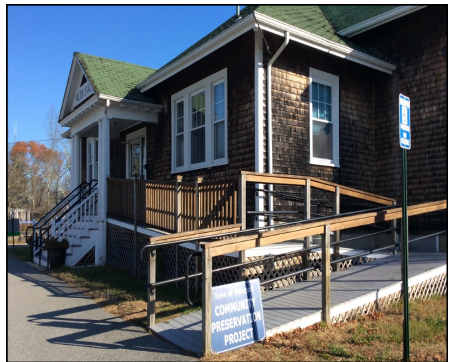
Fig. 1-1 CPA funded Town Hall Annex ADA Ramps
