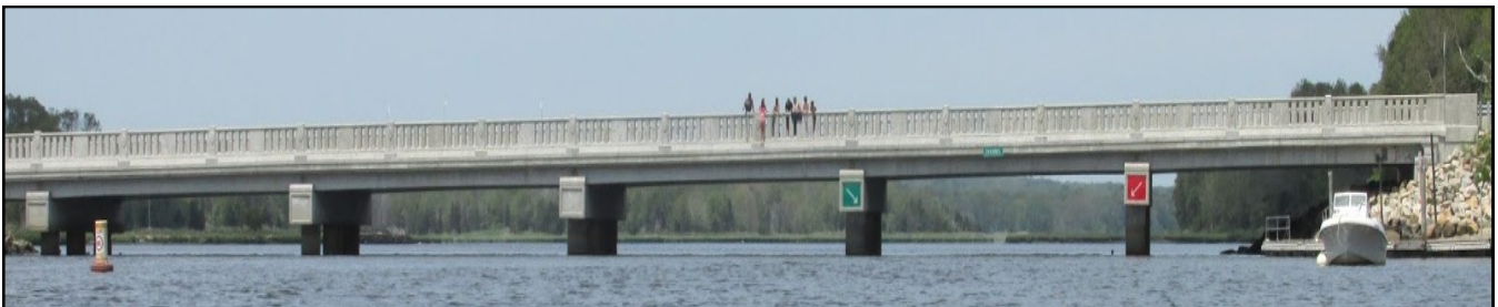
Fig. 7-6 Hix Bridge on Hix Bridge Road
