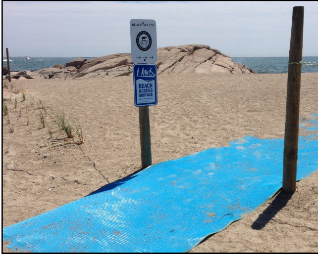
Fig. 8-4 Beach Avenue Mobi-mat installation.
