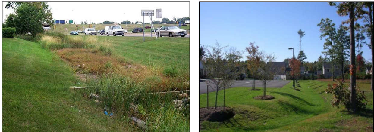
Figure 12. Example of BMP – Wet and Dry Swales
