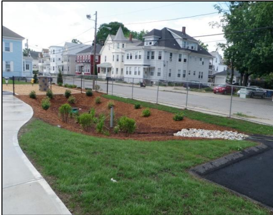
Figure 10. Example of BMP - Bioretention Basin
