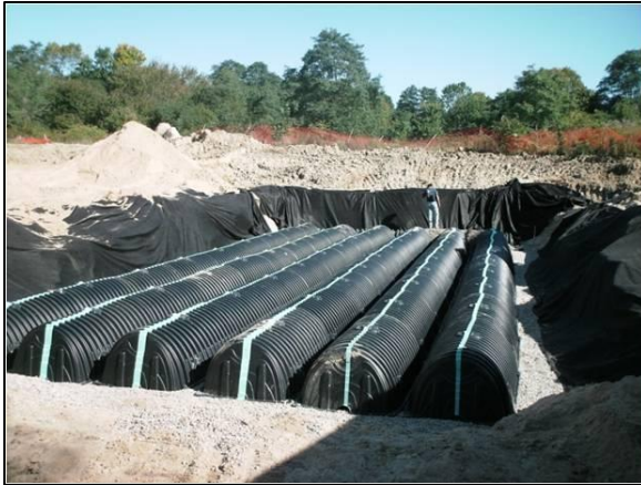
Figure 11. Example of BMP - Underground Infiltration
