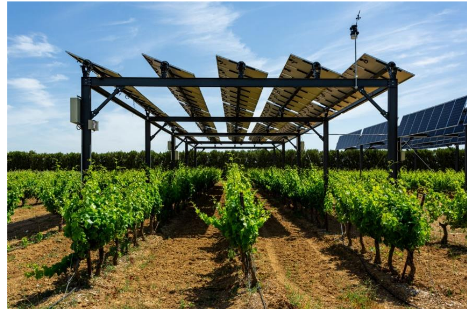
An agrivoltaic system demonstrating a vineyard underneath solar panels. Source: PV Magazine.
