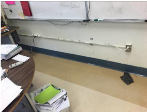
Typical wall receptacle added in classroom
