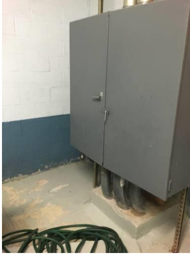
Automatic Transfer Switch
