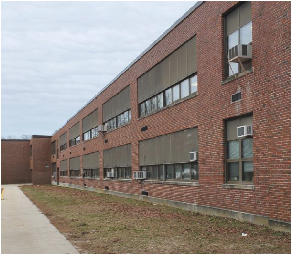
Exterior facade: The brick building envelop appears to be in fair condition with minor deterioration. The lack of central air is made obvious by the numerous air conditioner units on the facade.
