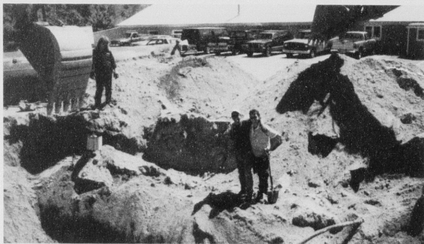
Removal of Underground Storage Tanks Behind Police Department Garage
