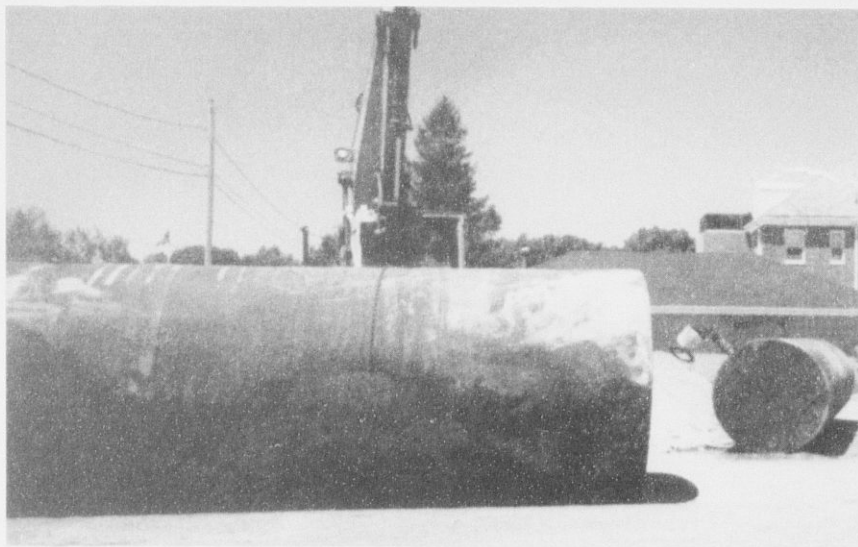
10,000, 4,000 & 500 Gallon Underground Storage Tanks Removed from Town Property
